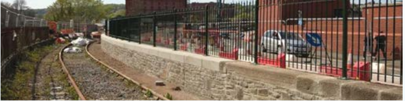
Plate 1 - Cumberland Road flood wall
