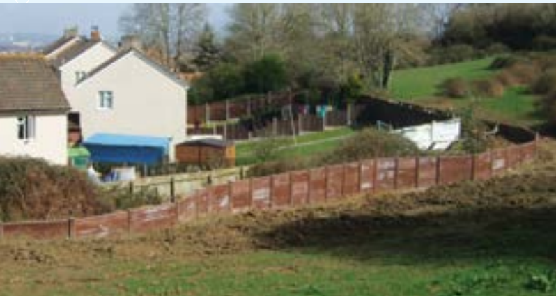
Plate 2 – Flood proof fencing in south Bristol
