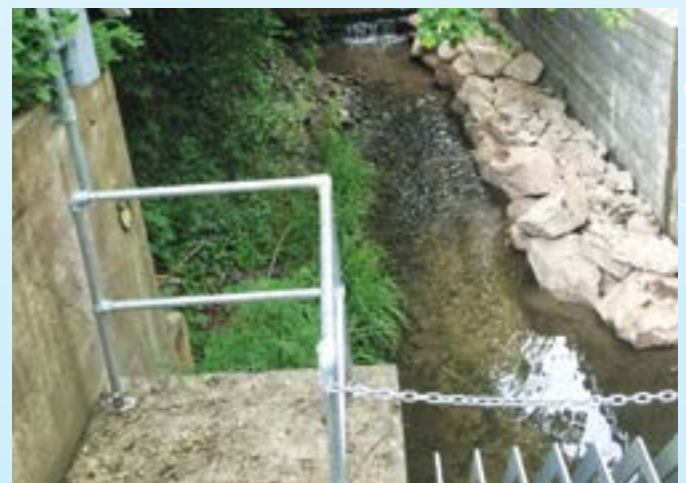
Plate 3 – The new Brislington Brook retaining wall reducing fluvial flood risk
